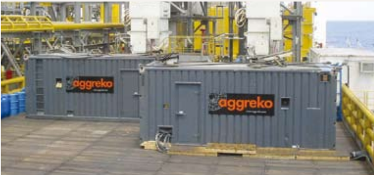
Containerised generators
